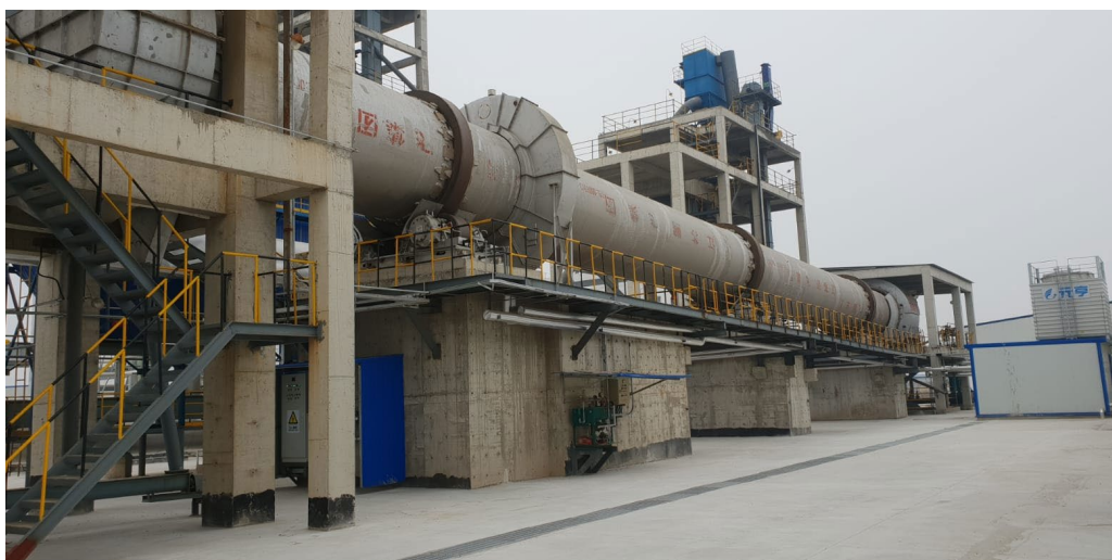
Figure 5: Direct Fired Rotary Kiln
